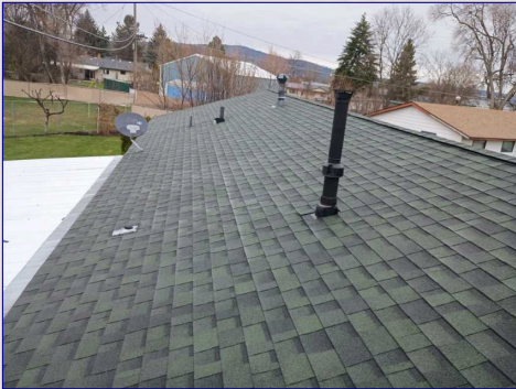
The Roof View
