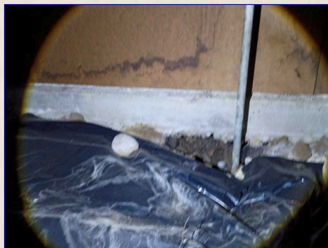
The main water pipe at front wall
