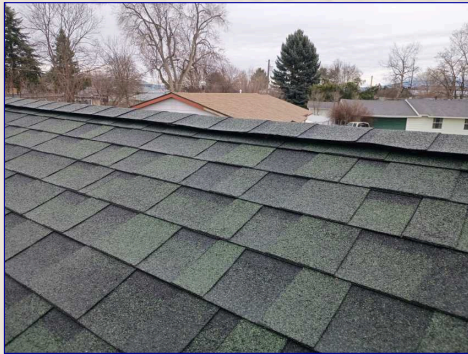
The Ridge Vent
