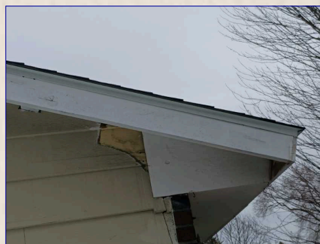
Flashing / Fascia View
