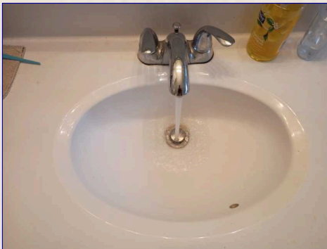
Sink faucet operating
