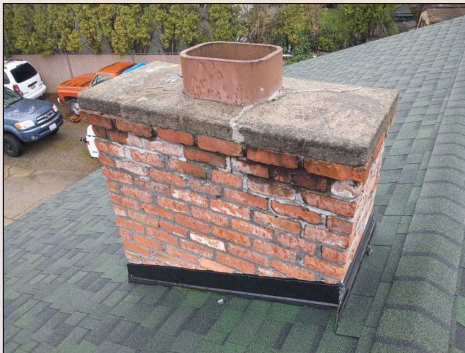
The Chimney Chase
