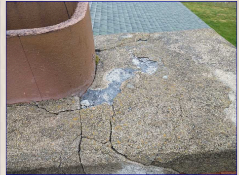
The Chimney Chase
