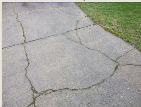
The Driveway View
