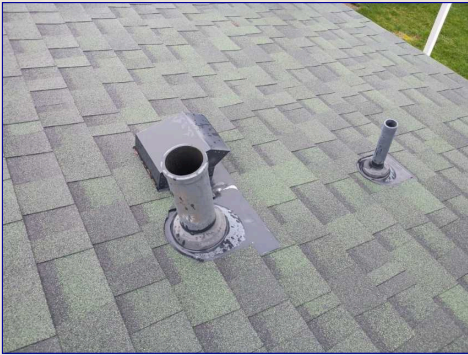
The Plumbing Vent(s)
