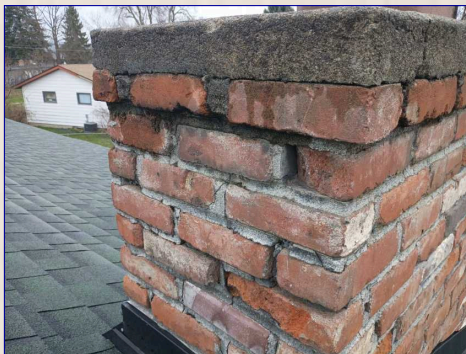
The Chimney Chase
