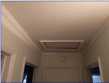
The Attic Access View
