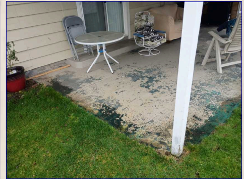
The Patio View
