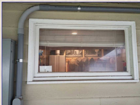
Laundry Room Window
