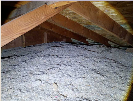
Attic Insulation View
