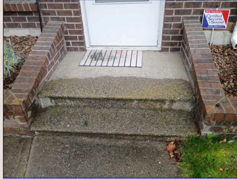
The Steps/Stoop View
