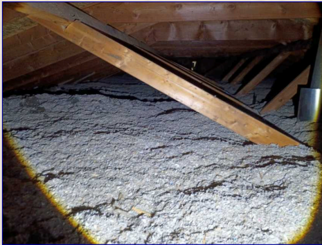
The Attic View
