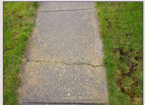
The Service Walk View
