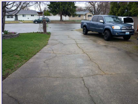
The Driveway View
