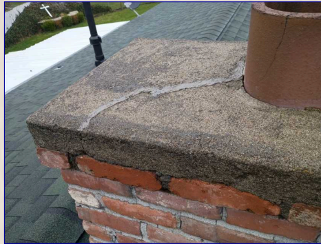
The Chimney Chase
