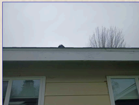
The Fascia View
