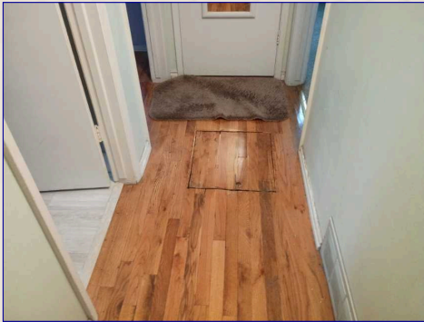
Crawlspace Access 1 Main Hallway
