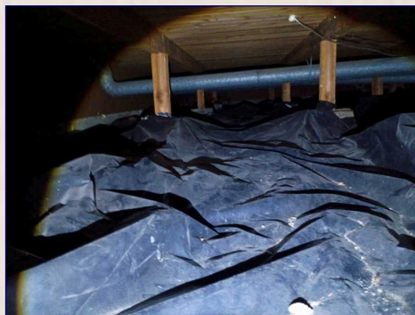
The crawlspace walls view
