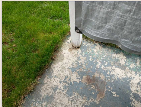
The Deck/Porch/Patio Cover View
