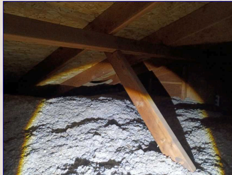
Attic Insulation View
