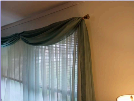
The ceiling/walls had cracking in various rooms. Recommend a licensed contractor repair as needed.
