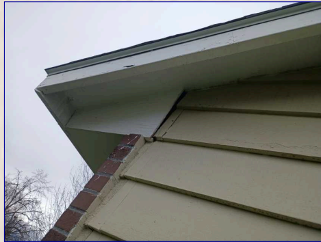
The soffit view.
