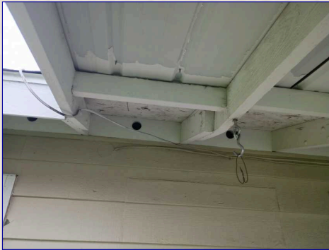
The Deck/Porch/Patio Cover View
