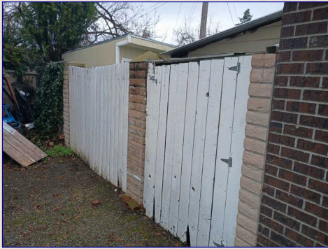
The Fence View
