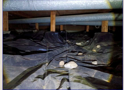
The crawl space floor
