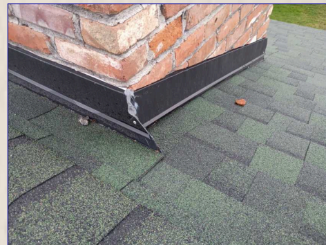
The Chimney Chase
