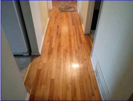
Main Hallway Flooring View
