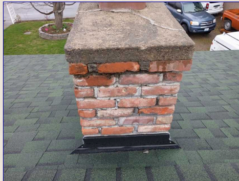
The Chimney Chase
