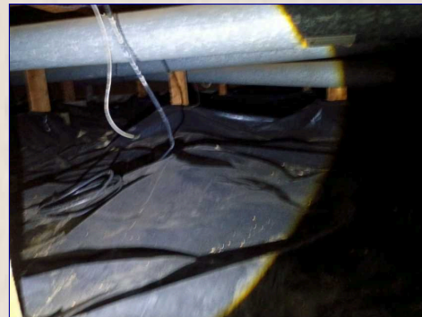
The crawl space floor
