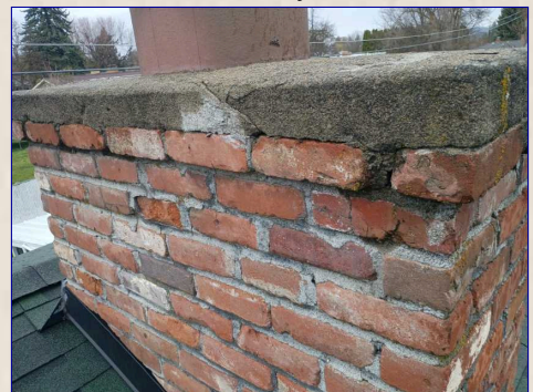
The Chimney Chase
