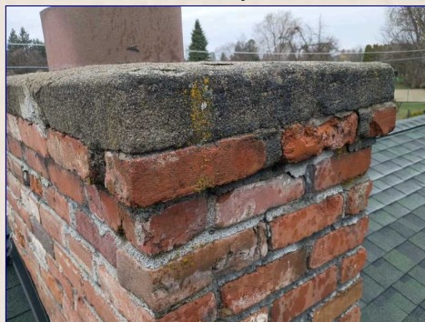
The Chimney Chase
