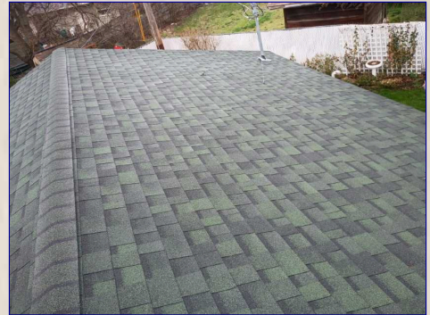
The Roof View
