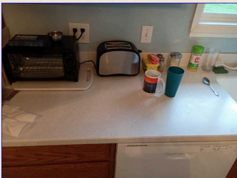
The caulk was missing dried or cracked.
