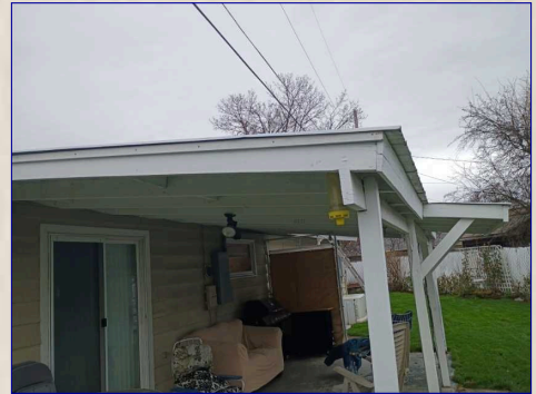
The Deck/Porch/Patio Cover View
