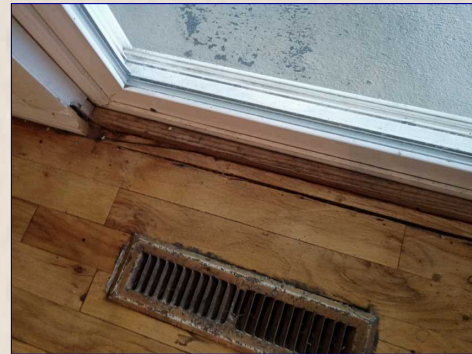
Sill at door 2 Entry in Dining Room
