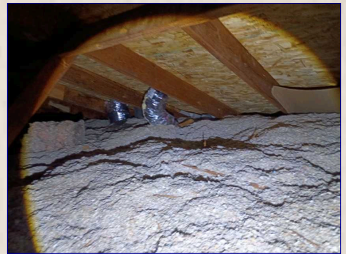
The Attic View
