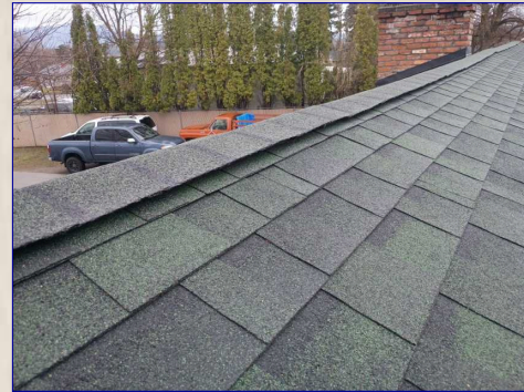
The Ridge Vent
