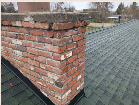
The Chimney Chase
