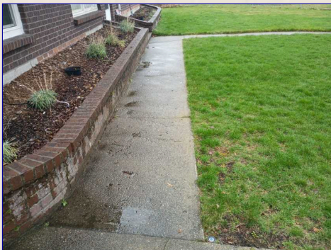
The Service Walk View
