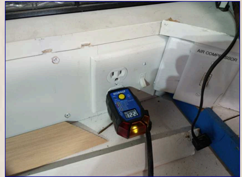
Electrical Receptacle Operating
