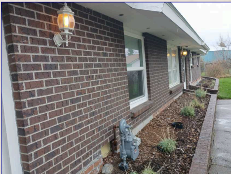
Brick veneer siding view
