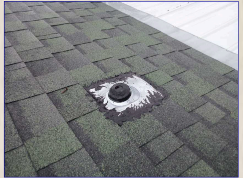
Previous Electrical Service Entrance
