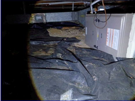
The crawl space floor
