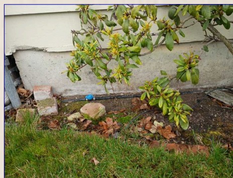
Foundation wall view.
