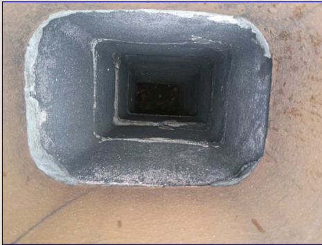
The Chimney Chase
