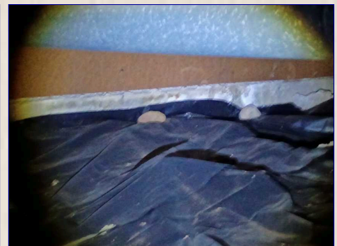
The crawlspace walls view
