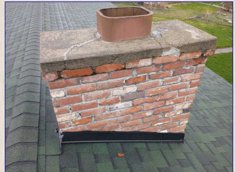
The Chimney Chase
