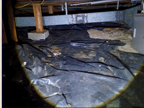
The crawl space floor
