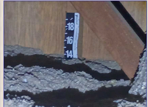
Attic Insulation View
